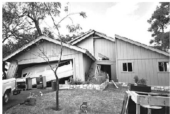
Figure 5 - San Simeon Earthquake, Dec. 22, 2003 This home slid 2 feet off its foundation due to inadequate nailing of walls to its sill plates.
