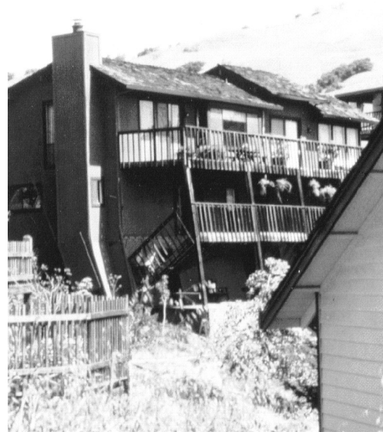
Figure 18 - This hillside home was built on an unbraced tall wall that failed.
