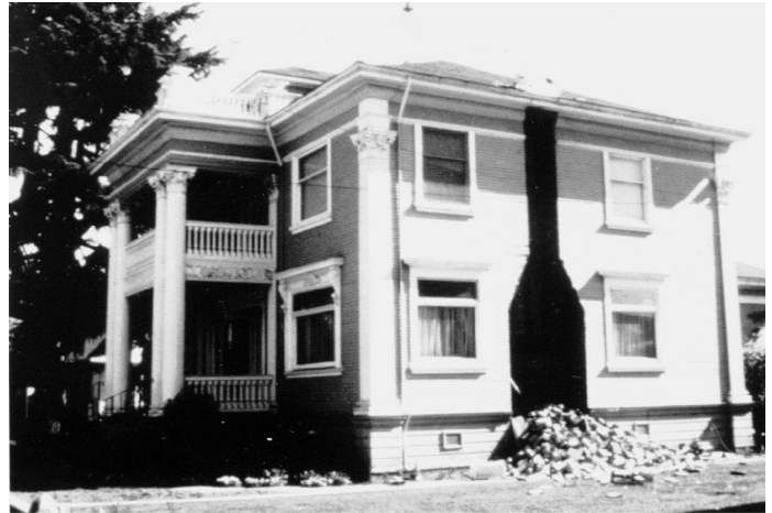
Figure 29 - This unreinforced chimney fell during a recent earthquake.
