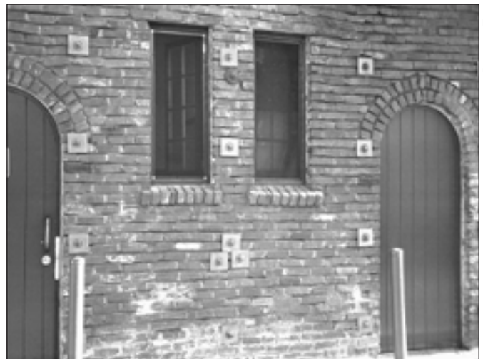
Figure 24 - Bolting of unreinforced masonry wall to steel frame on the inside.
