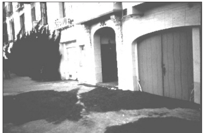
Figure 36 - Loma Prieta Earthquake, October 17, 1989. Lateral spreading, liquefaction and sand boils caused extensive damage in the Marina District of San Francisco, about 60 miles away from the epicenter.
