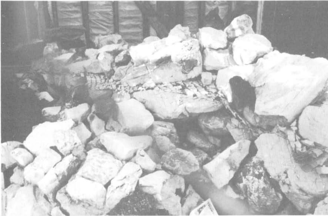
Earthquake Damage: 1994, Northridge, California Photo Credit: Robert Reitherman
