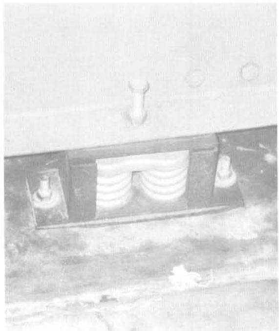
Chiller mount with no uplift resistance and insufficient or no shear resistance. Photo Credit: Wiss, Janney, Elstner Associates, Inc. Schematic Upgrade Detail: See Detail U32, Air Compressor
