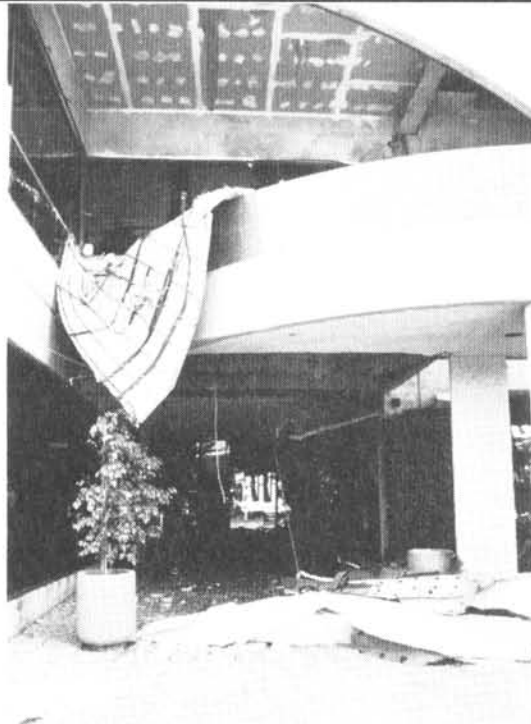
Failure of heavy stucco soffit at building entrance Earthquake Damage: 1994, Northridge, California Photo Credit: Robert Reitherman
