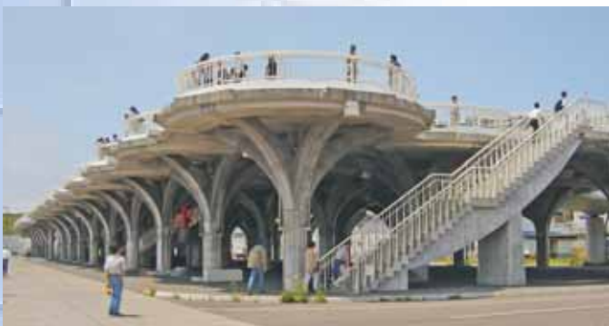
Elevated platform used for tsunami evacuation that also serves as a high-elevation scenic vista point for tourists. Okushiri Island, Japan. Photo courtesy of ITIC.
