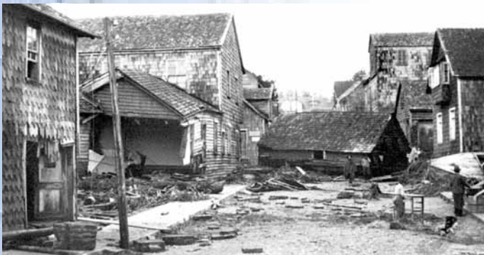
Damage caused by the 22 May 1960 Chilean tsunami. Photo courtesy of Ilustre Municipalidad de Maullin, USGS Circular 1187.
