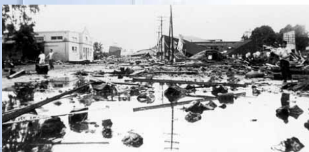
Destruction along the waterfront of Hilo, Hawaii from the Pacific-wide tsunami generated off the coast of Unimak Island, Aleutian Island, USA on 1 April 1946.
