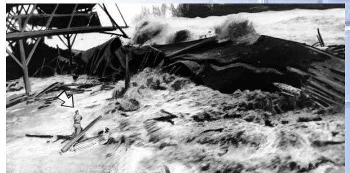
Destruction of Hilo Harbor, Hawaii, 1 April 1946. The tsunami generated off the coast of Unimak Island, Aleutian Islands raced across the Pacific, coming ashore in Hawaii less than five hours later. Photo courtesy of NOAA.
