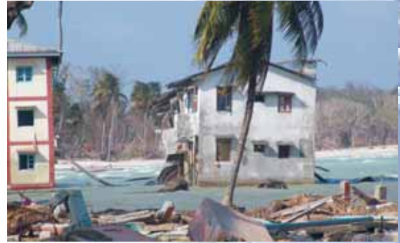
The 26 December 2004 earthquake resulted in 1.2 m of land subsidence in the Car Nicobar, Nicobar Islands, India leaving houses that were once above sea level now permanently submerged. Photo courtesy of ICMAM, Chennai, DOD, India.
