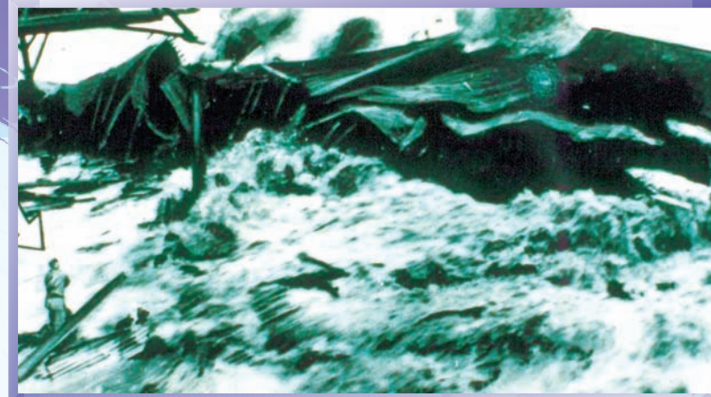
Hilo Harbor, Hawaii, April 1, 1946, Aleutian Islands earthquake. Photo taken from the vessel Brigham Victory of tsunami breaking over Pier 1. The gentleman on the left did not survive. (NOAA)
