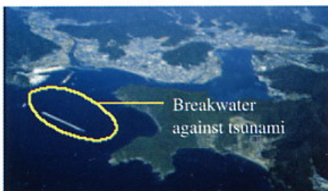
(9) Constructing Break Water
