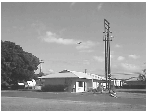
Geostationary satellite antennas (left, partially hidden behind tree) and VHF radio antennas (right, at top of tower) make up part of PTWC's many communications
