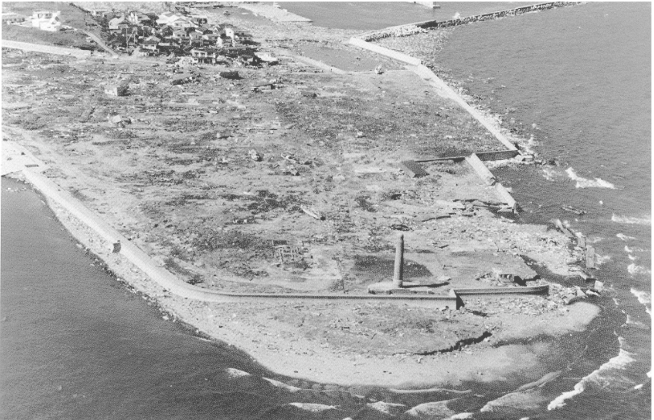
Massive destruction in the town of Aonae on Okushiri Island, Japan caused by the regional tsunami of July 12, 1993.
