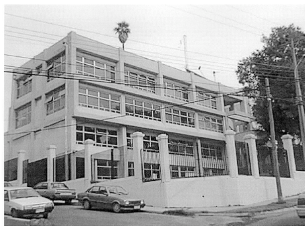
Headquarters of the Chilean Tsunami Warning System (SNAM) operated by the Hydrographic and Oceanographic Service of the Chilean Navy is located in Valparaiso.
