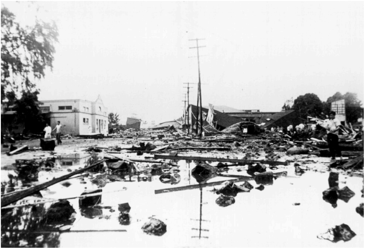
Destruction along the waterfront of Hilo, Hawaii from the Pacific-wide tsunami generated off the coast of Unimak Island, Alaska, USA on April 1, 1946.
