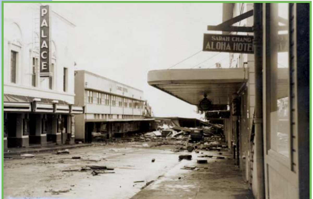
Tsunami damage and debris on Hilo Street following the April 1, 1946 tsunami.
