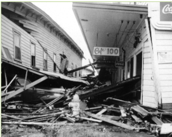
Café 100 damaged after the 1946 tsunami.
